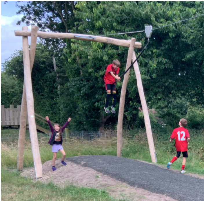
Children enjoy the new zip wire. The frame is made from hardwood timber, there are steel ground anchors, and the runway has safety surfacing.
